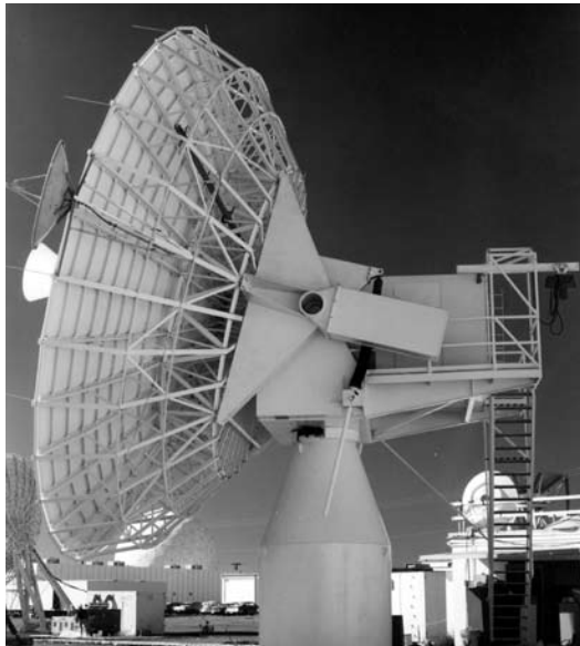
Many large radar antennas at research and National Weather Service installations turn on Rotek Series 15,000 Wire-Race slewing rings.
